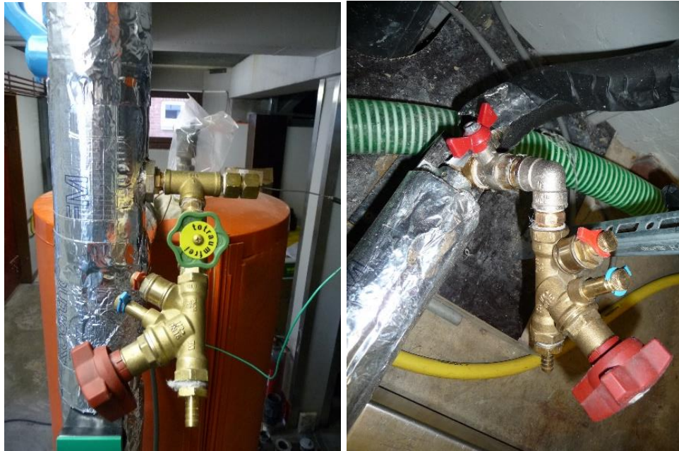
Figure 3 – Sampling points near the test tank : (left) temperature probe in the T-piece and sampling tap upstream a flow regulation valve on the departure pipe. (right) Sampling valve upstream of a flow regulation valve on the recirculation loop.
