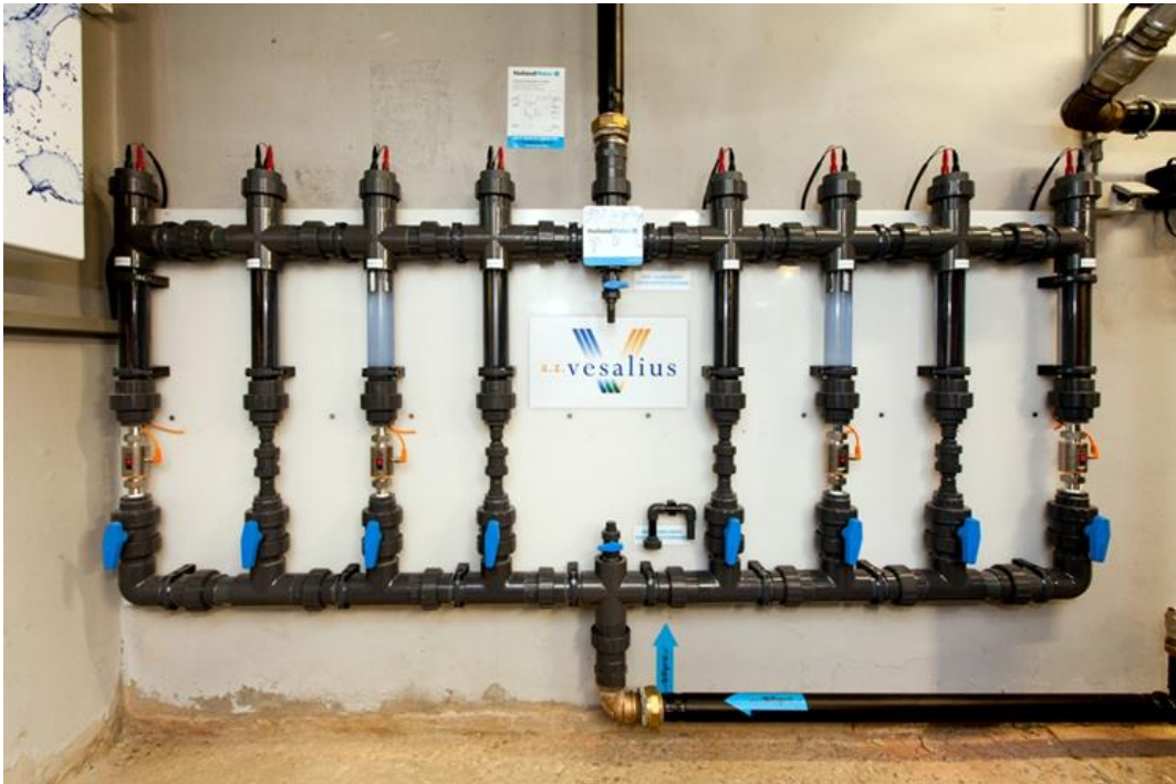
Figure 7- The Bifipro equipment (CSI unit) with 6 copper and 2 silver ionisation cells. The input is located in the centre under the ionisation cells
