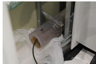
Photograph 2 – Survey of calcified urine in horizontal branch drainpipe using Industrial-Videoscope
