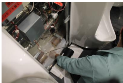
Photograph 2 – Survey of calcified urine in horizontal branch drainpipe using Industrial-Videoscope
