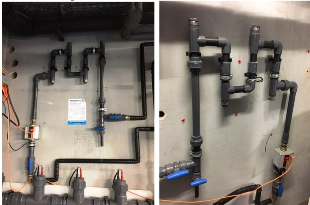
Figure 7- The Bifipro equipment (CSI unit) with 6 copper and 2 silver ionisation cells. The input is located in the centre under the ionisation cells
