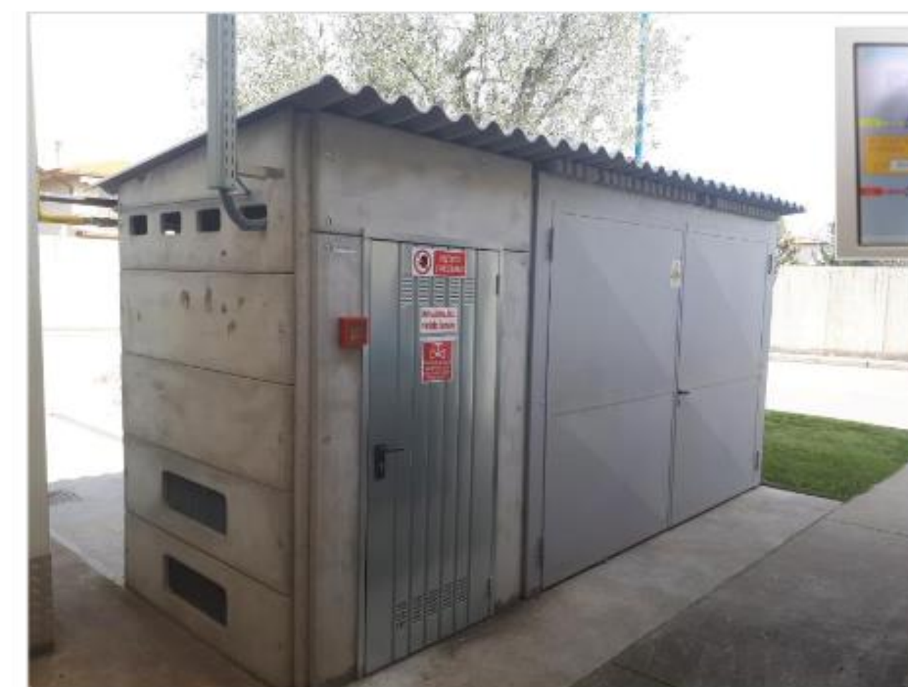
H2 bottles Storage and mixing station
