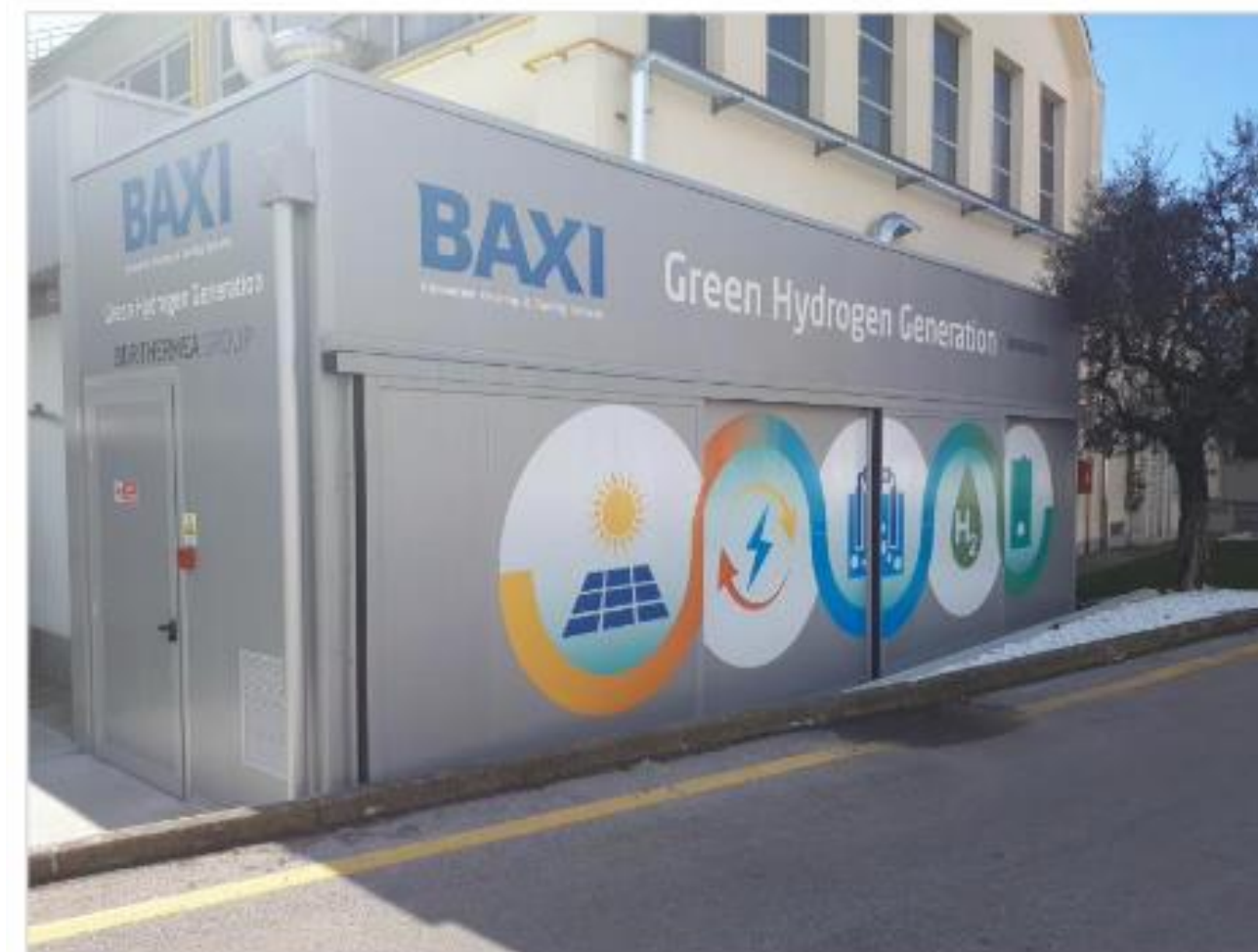
Electrolysers for Green Hydrogen (25 m 3 /h)
